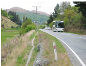
Unsafe pedestrian and cycle access beside the road to Arthur's Point
